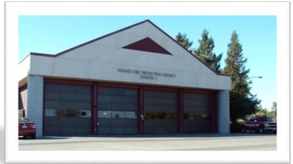
Station 61 7025 Redwood Blvd
