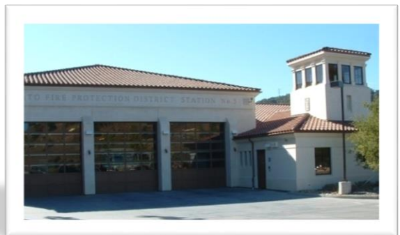
Station 65 5 Bolling Drive
