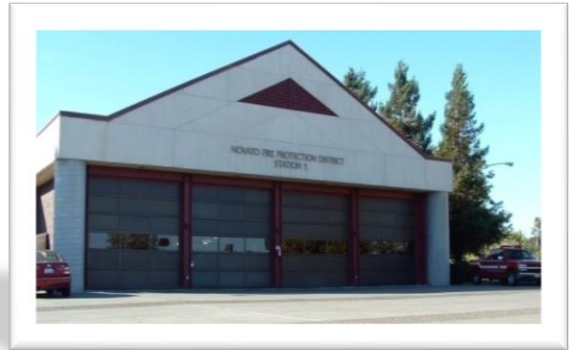
Station 61 7025 Redwood Blvd
