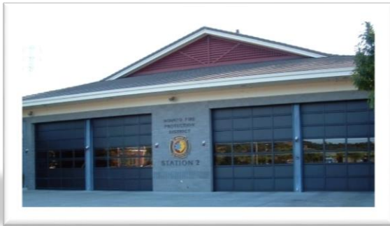
Station 62 450 Atherton Avenue
