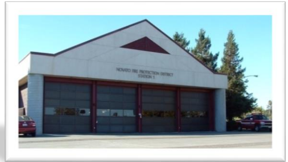
Station 61 7025 Redwood Blvd
