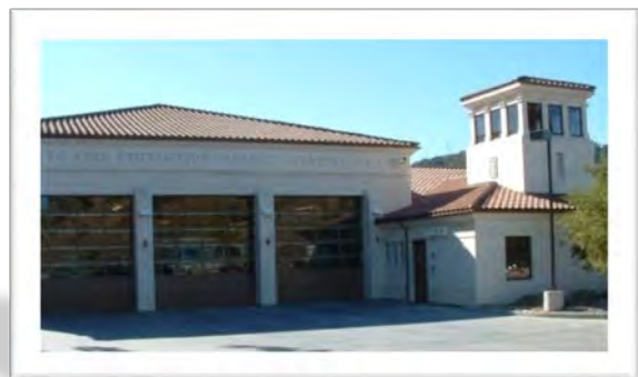
Station 65 5 Bolling Drive
