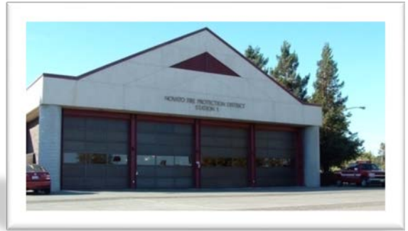
Station 61 7025 Redwood Blvd
