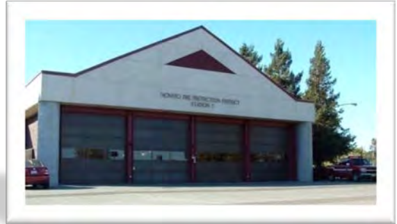
Station 61 7025 Redwood Blvd
