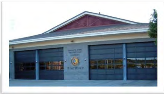
Station 62 450 Atherton Avenue
