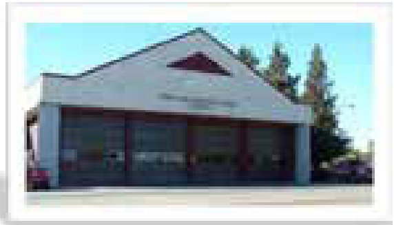
Station 61 7025 Redwood Blvd
