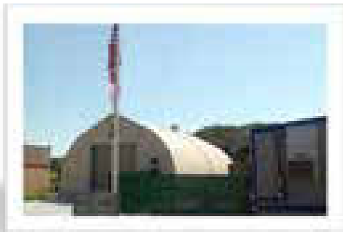
Station 64 105 Roblar Drive
