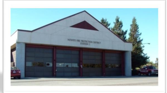
Station 61 7025 Redwood Blvd
