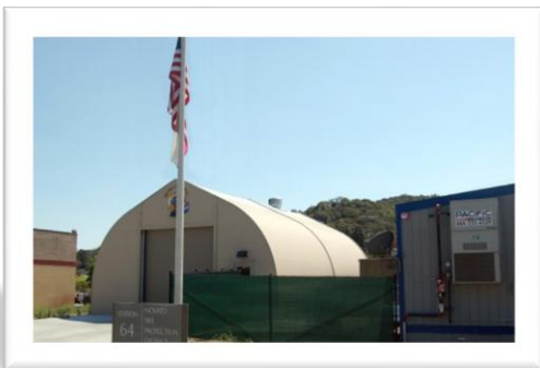
Station 64 105 Roblar Drive
