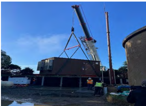
Muir Beach shelter being lifted into place.
