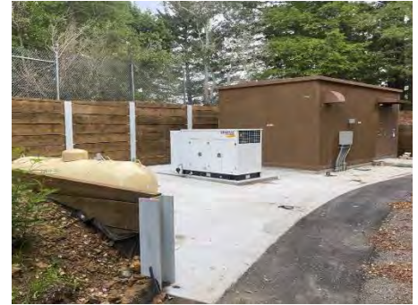
Mill Valley water tank site.
