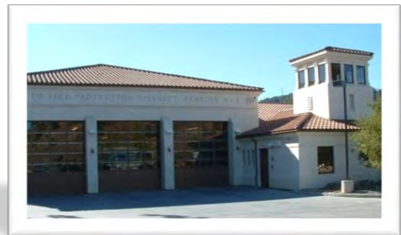
Station 65 5 Bolling Drive
