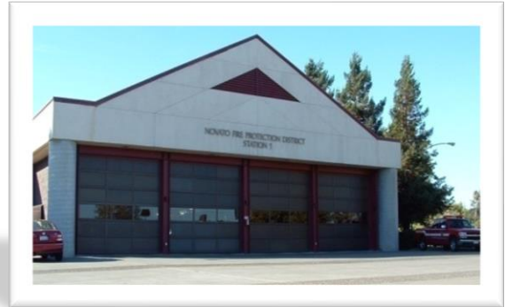
Station 61 7025 Redwood Blvd
